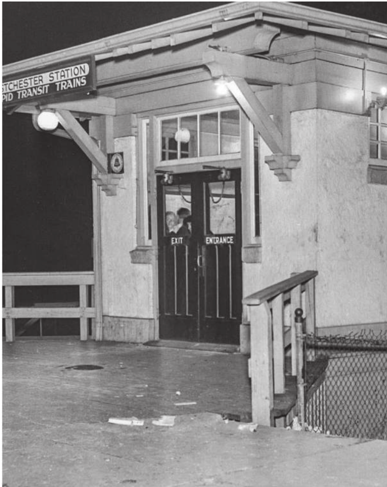
Former Roosevelt Station
