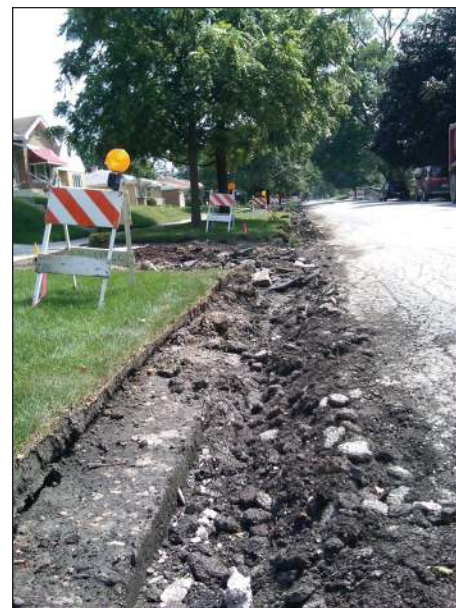
Curb and apron removal
